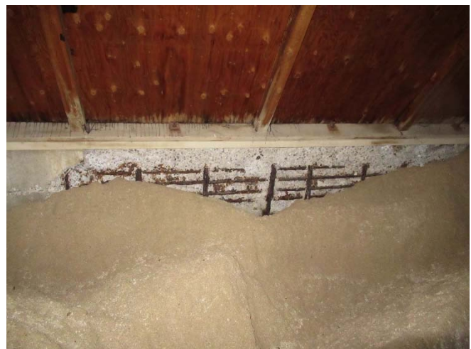
Photo 31: Delaminated (corrosion damaged) sand dome concrete foundation walls with exposed reinforcing steel.
