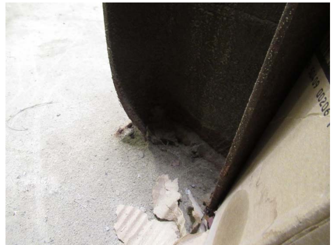
Photo 5: Impact damage to a steel column.
