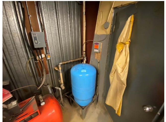
Photo 22: Incoming line from well and expansion tank.
