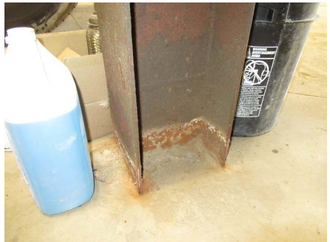
Photo 2: Corrosion at the base of a column.
