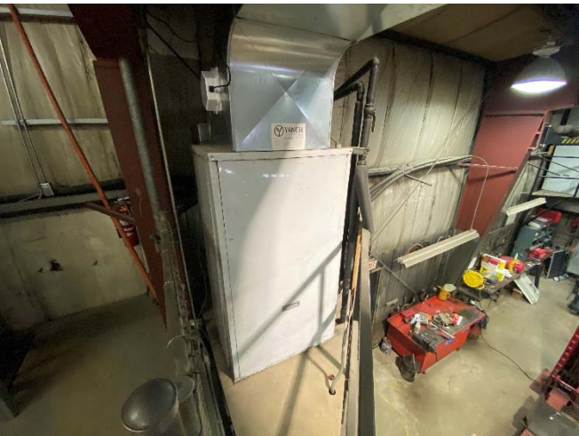
Photo 18: 6 ton ground source heat pump unit.
