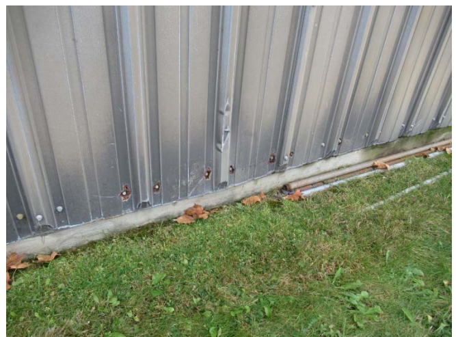
Photo 8: Corrosion and impact damage at bottom of metal cladding on the north elevation.
