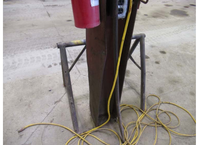
Photo 4: Impact damage to a steel column.
