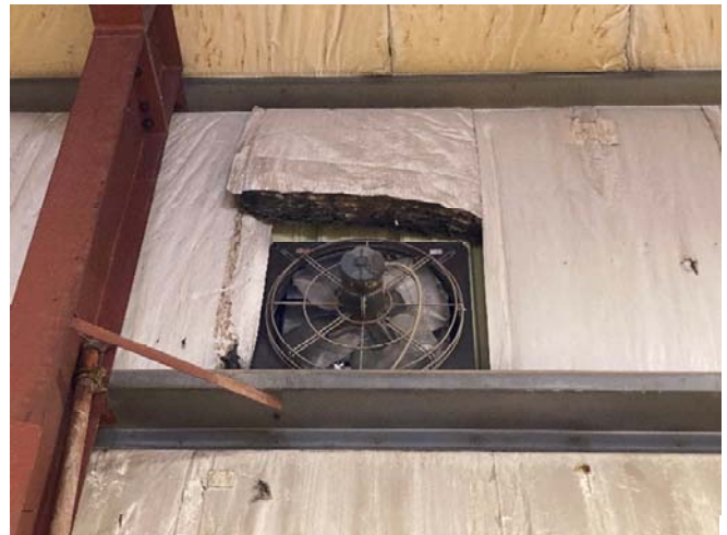
Photo 21: Typical wall mounted exhaust fan.
