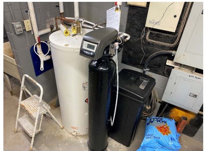
Photo 23: Hot water heater and water softener.
