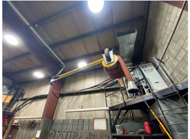
Photo 20: Truck exhaust system.
