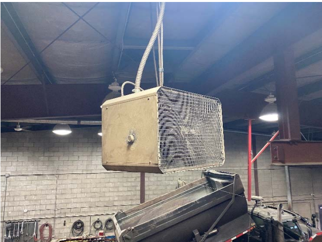
Photo 19: Supplemental electric unit heater.
