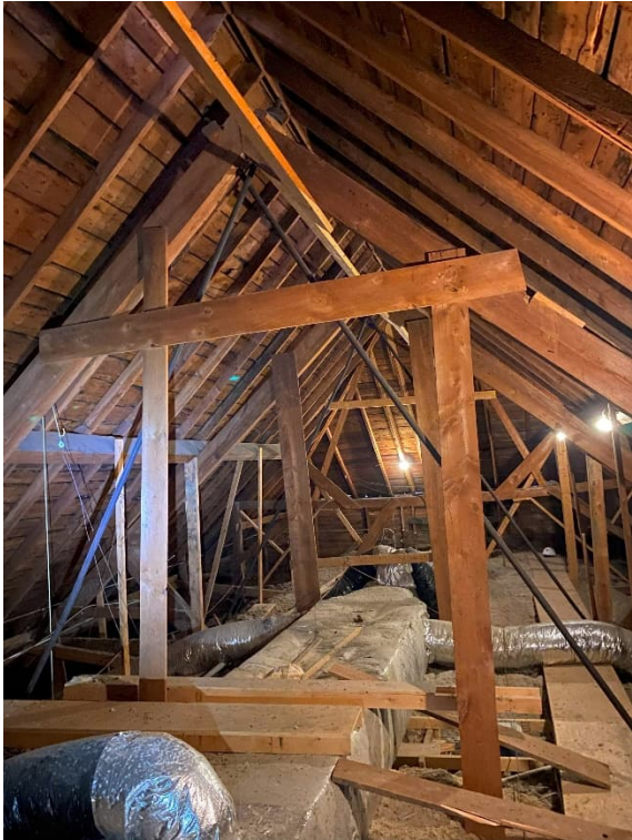
Photo 12: Trusses and Rafters in the Attic (Main Roof)
