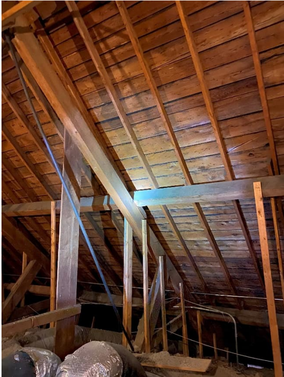
Photo 10: Trusses and Rafters in the Attic (Main Roof)
