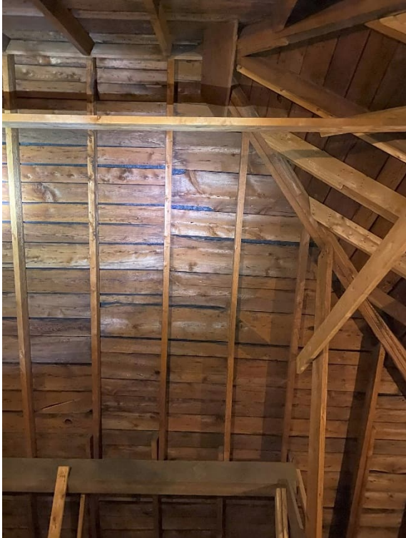
Photo 13: Splitting Wooden Planks at Main Roof
