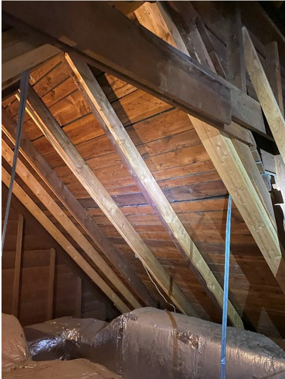
Photo 17: Rafters in the Attic (Low Roof)
