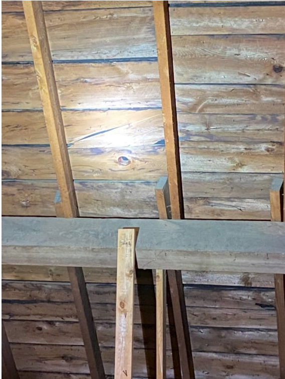
Photo 14: Splitting Wooden Planks at Main Roof
