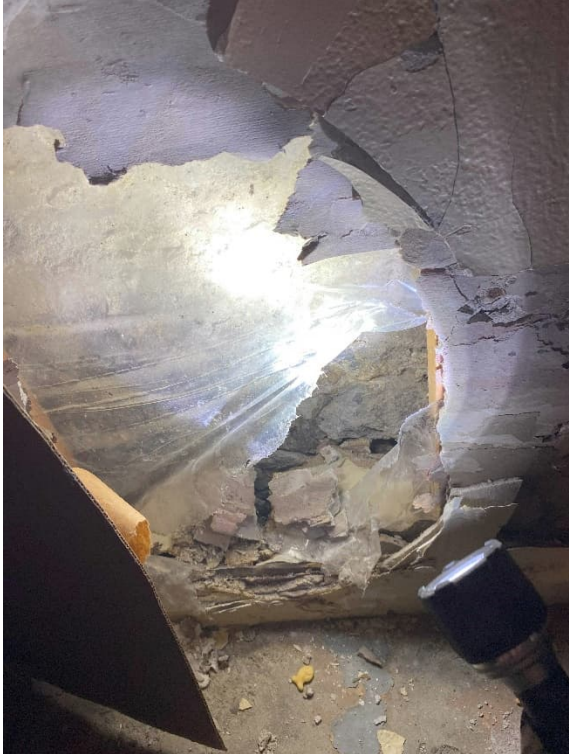
Photo 23: Exposed Foundation Wall
