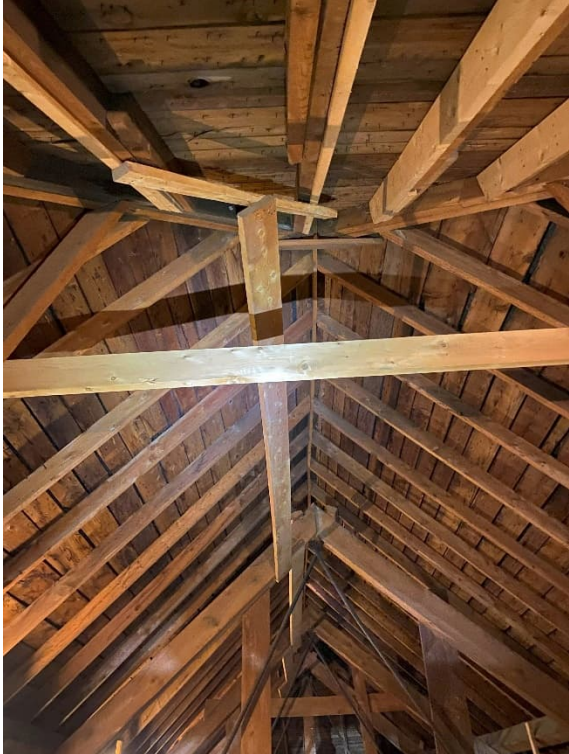
Photo 9: Trusses and Rafters in the Attic (Main Roof)
