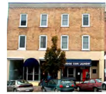
Figure 29 Asymmetrical window and storefront proportions.
