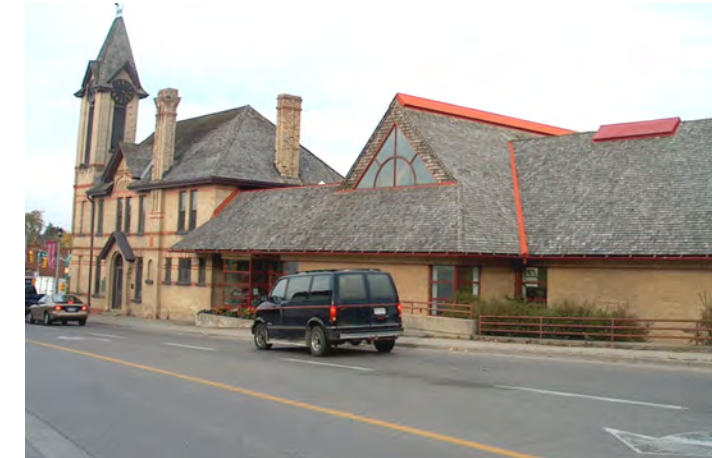
Figure 43 Roof pitch, massing, and material of this addition to the Joseph Gould Library allow this modern building to fit well with its predecessor.
