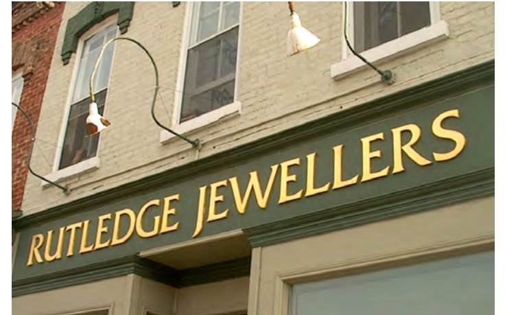
Figure 20 When storefront signage is located on the entablature above the storefront, opportunities for traditional lighting exist.
