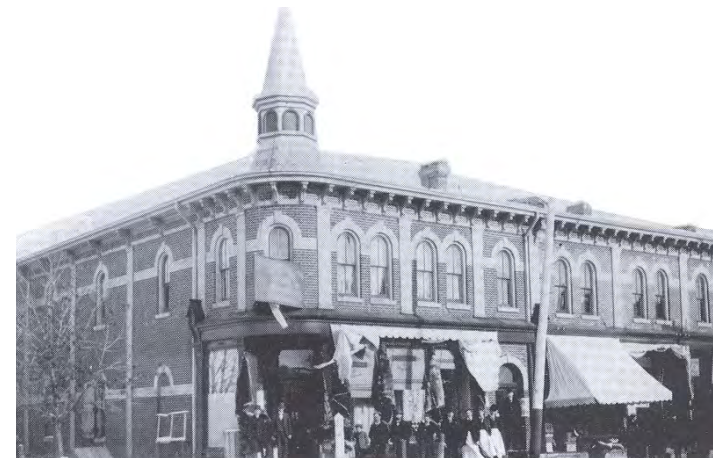
Figure 41 Henry's Department Store, which formerly resided on the north-east corner of Brock and Spruce Street, burned down in 1902 leaving the site empty for the construction of the post office pictured on the right.
