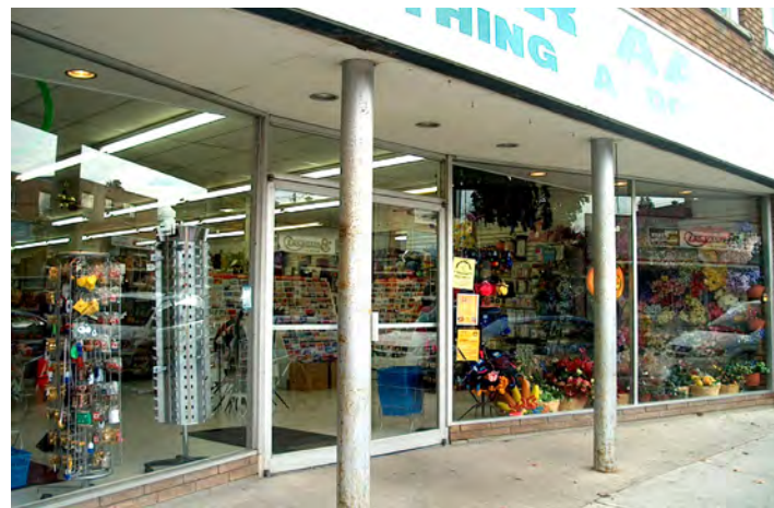
Figure 16 Several contemporary storefronts along Brock Street exhibit only some of the attributes of a desirable storefront design including in this example, a recessed entry.
