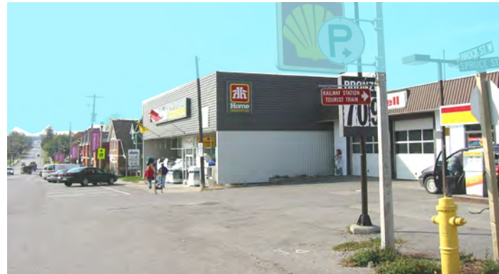
Figure 25 The building façade does not meet the required setback.
