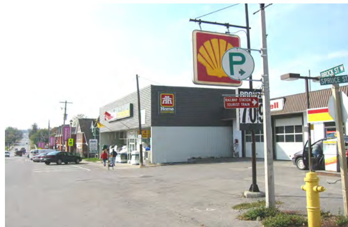
Figure 56 Improved sidewalks, curb lines and drive access into the Shell station should be considered as part of the Region's streetscape improvements.
