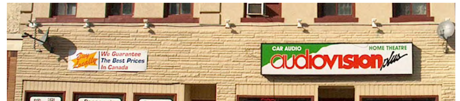
Figure 45 Back-lit sign boxes applied to historical building façades detract from the overall building appearance.
