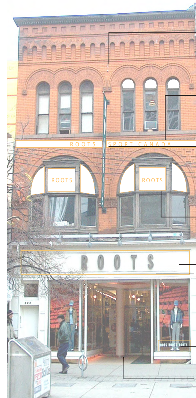
Figure 52 Storefront signage examples.
