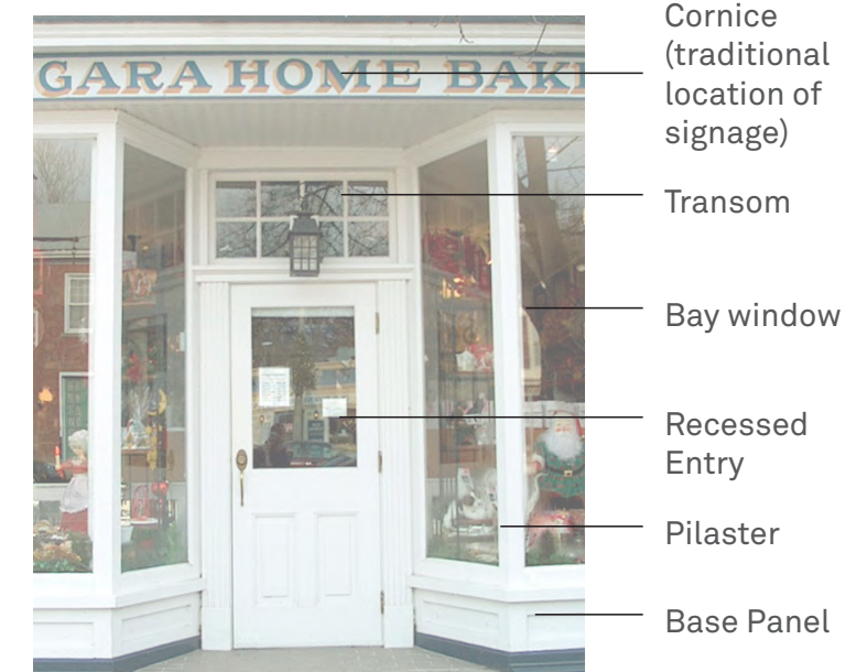
Figure 14 Parts of traditional storefront.
