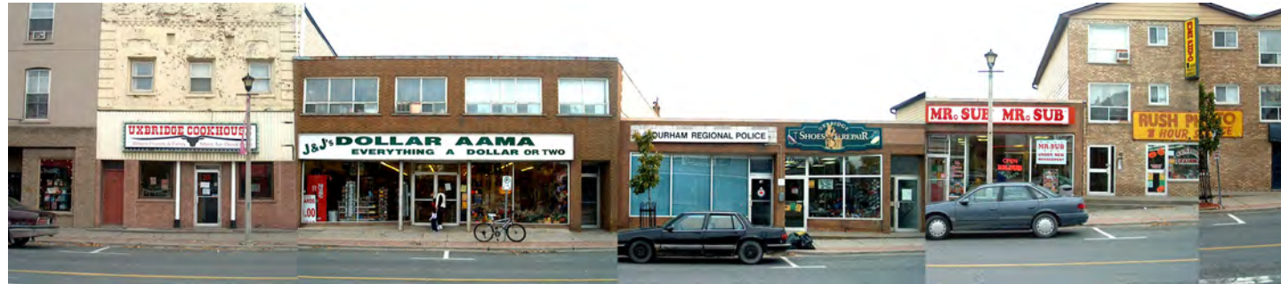
Figure 46 Back-lit sign boxes often deteriorate the original storefront frame due to improper flashing details.
