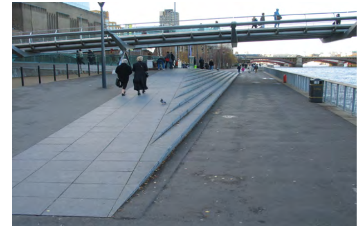
Figure 64 The combined stair and ramp along the Thames handily manipulates change in grade in two directions. This same site condition exists along Brock St. and needs to be resolved as part of the upcoming streetscape reconstruction.
