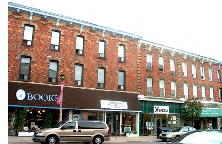
Figure 9 The 'original' commercial building block located between Bascom and Main Streets exhibits the Italianate 1:2 height to building width ratio.
